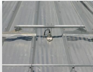
BRK1 & 2 roof support bracket for radius cables 35' - 50' in length.
