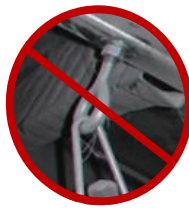
Bad Eyebolt Installation
