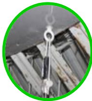
Good Eyebolt Installation
