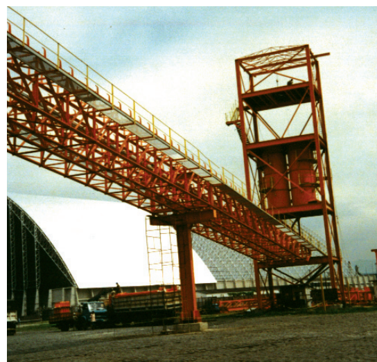
Metal structure for the flow scale
