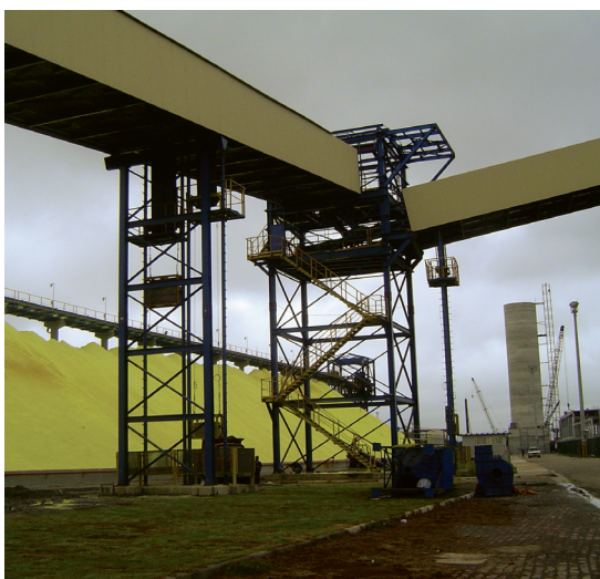
Metal structure with special painting for sulfur
